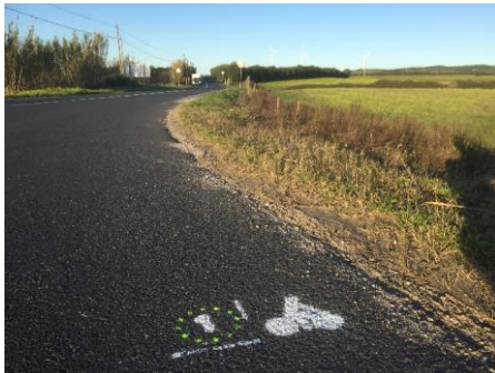
Example of road marking on EuroVelo 1 in Portugal, using the EuroVelo route information panel and a cyclist icon. In this example, the marking should be sharper.
