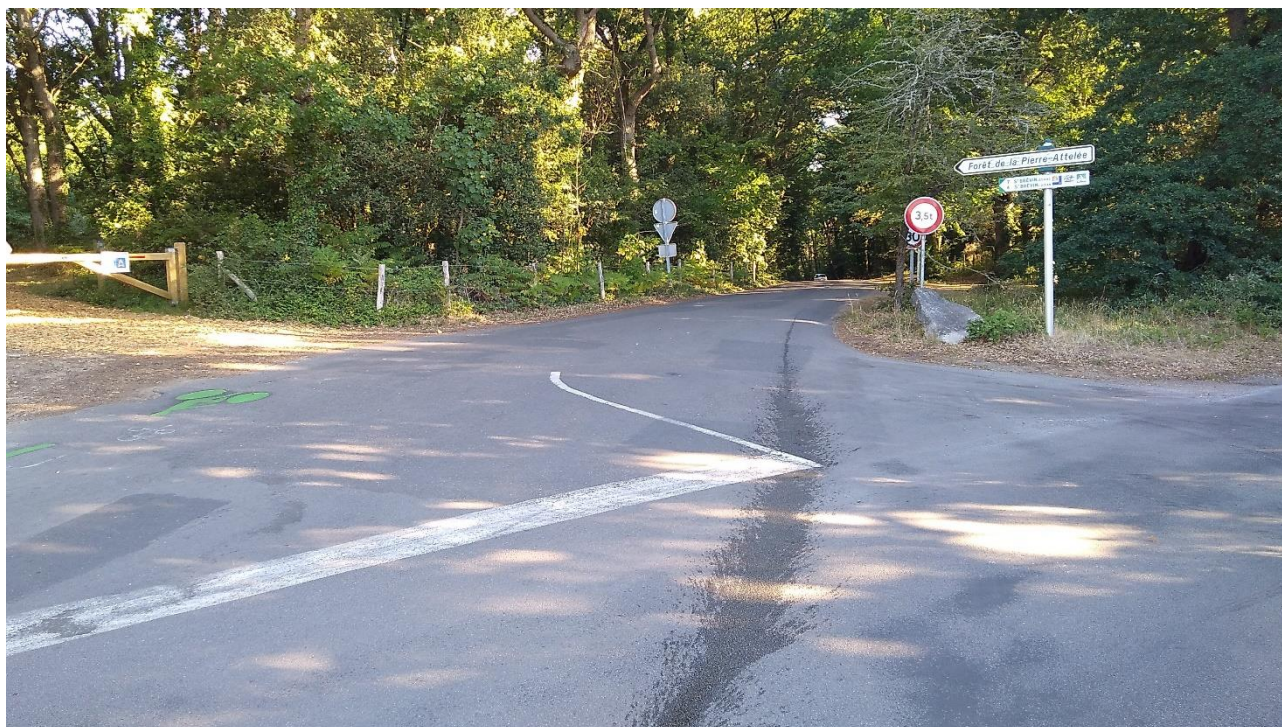
Confusing sign placement – indicates turn to the left, but there are two roads to the left. Which one to take? This can be resolved with a confirmation sign or an advance notice sign with a diagram of the crossing.
